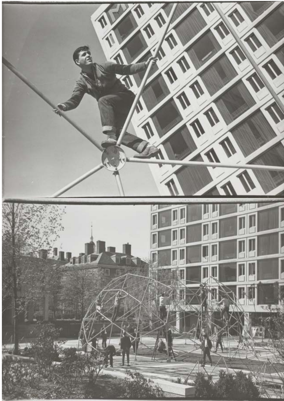
Caption: Lev Senior, playwright Blair Brown '62 scaling the dome; Erecting RB Fuller's geodesic dome in the courtyard. May 26, 1962.
